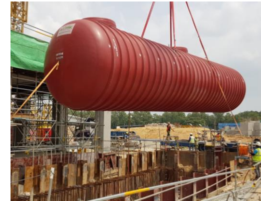
Fibre Reinforced Plastic Double Wall UL 1316 Fuel Tanks & BS Steel Single/Double Wall Tanks
