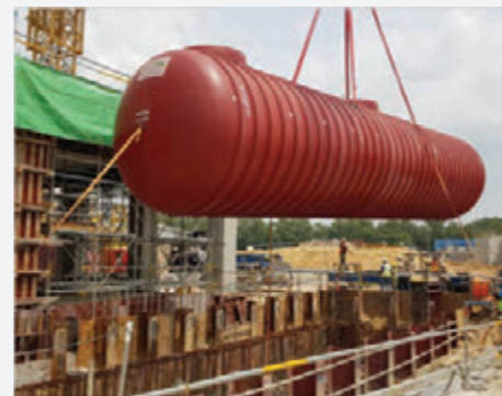
Bulk Diesel Storage Tank (Double Wall FRP) Capacity: 4,000 litres to 130,000 litres
