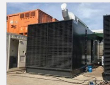
Acoustic Outdoor Generator Enclosures
