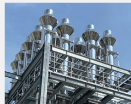
Double Walled Stainless Steel 304/304L or 316/316L Generator Exhaust Stacks
